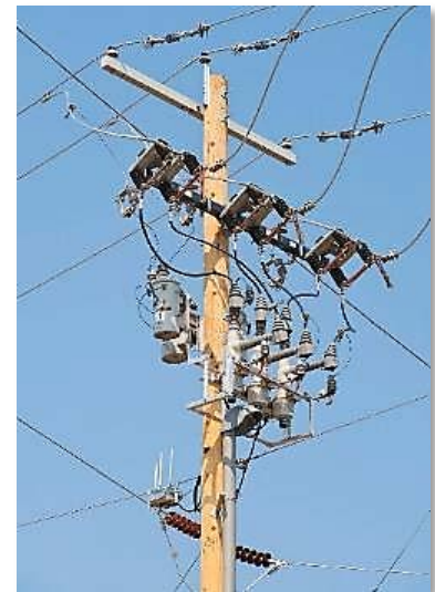
Figure 20. Dry Land Mode Device: Viper Recloser
