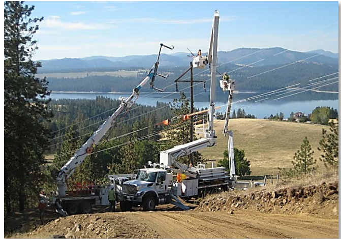
Figure 29. Addy-Gifford Steel Pole Replacement Work
